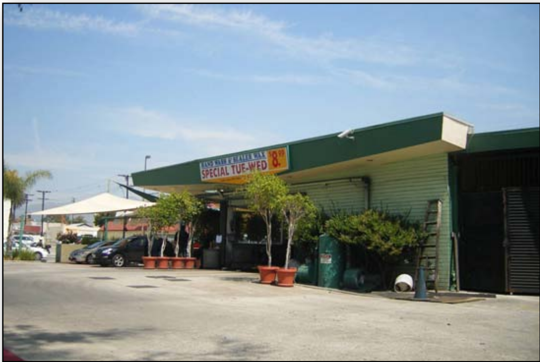
West elevation (San Fernando Road)
