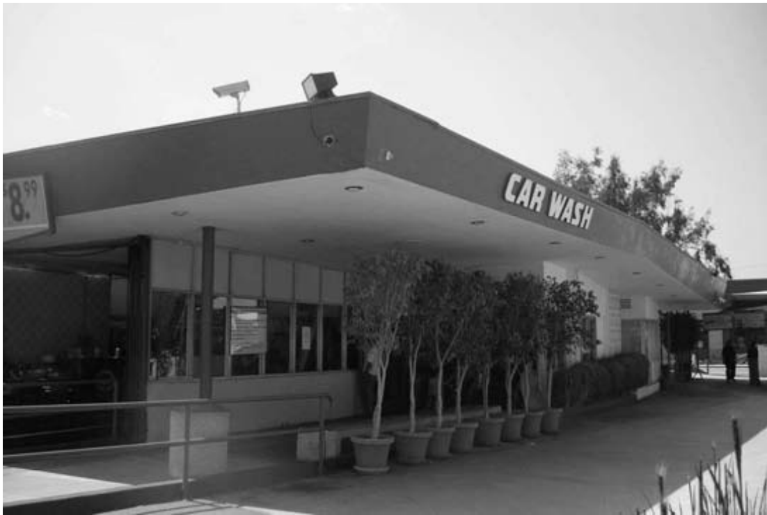
9. Corner, east and north elevations
