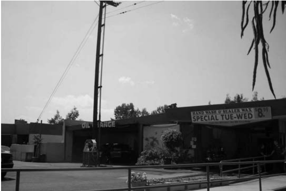
11. East elevation (facing Central Avenue)
