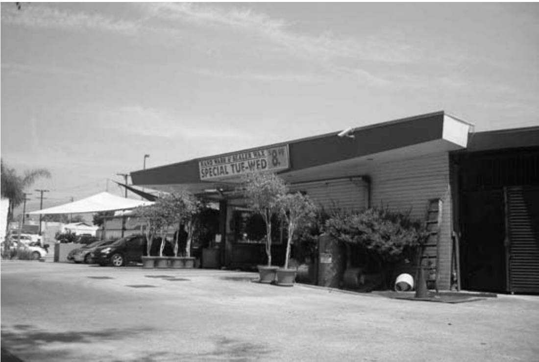
2. West elevation (San Fernando Road)
