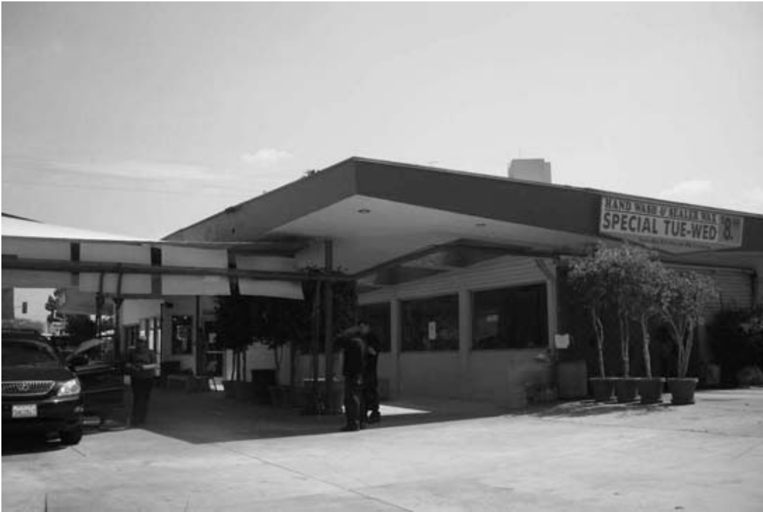
5. Corner, north and west elevations
