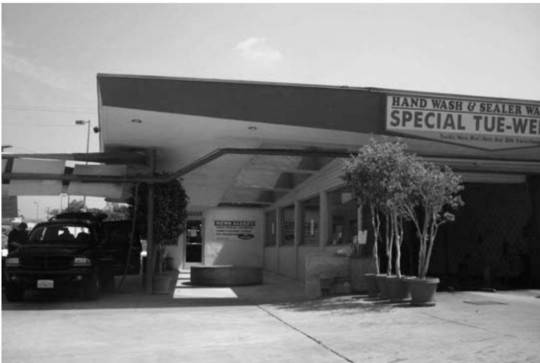
4. Corner, north and west elevations
