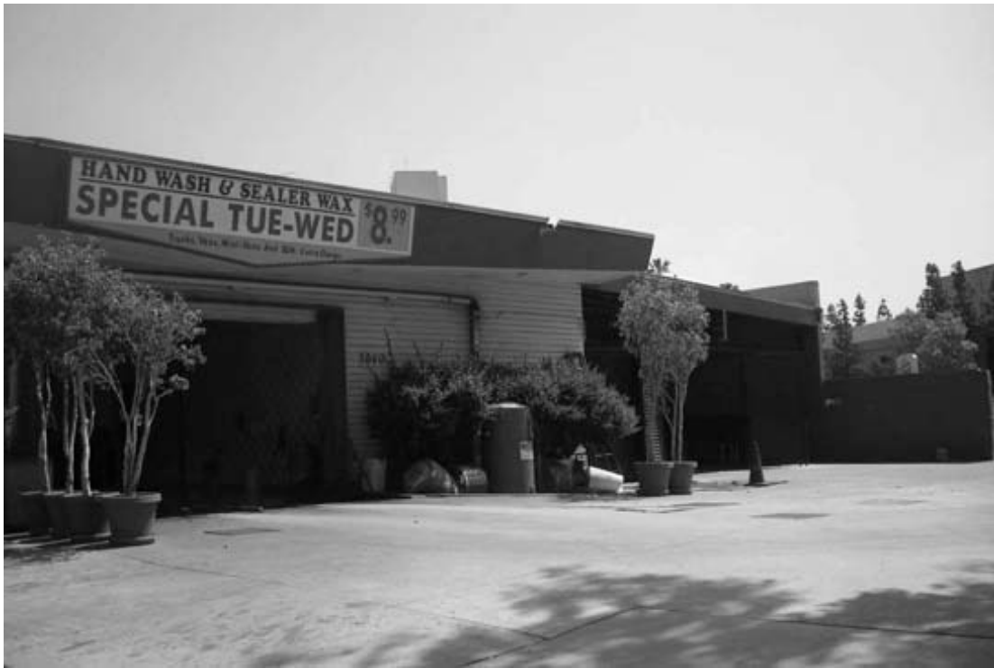
3. West elevation (San Fernando Road)
