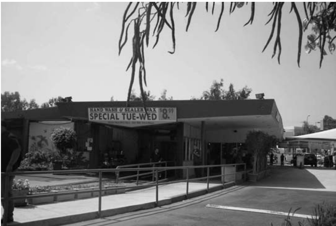
10. East elevation (facing Central Avenue)
